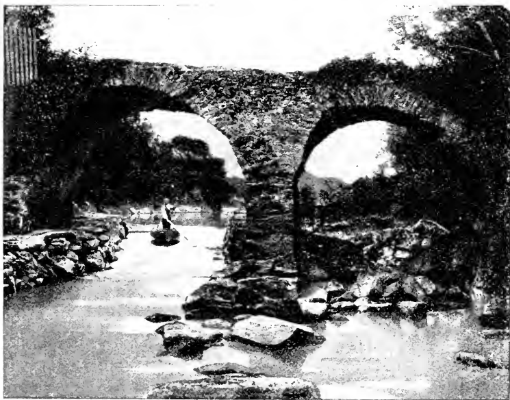
OLD WIER BRIDGE, KILLARNEY.
